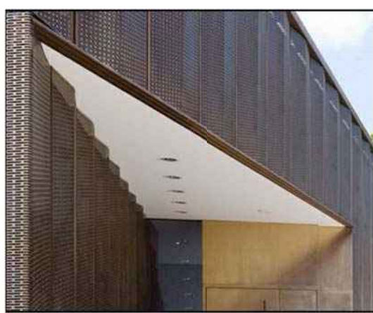
8. FIBRE CEMENT SOFFIT LINING PAINT FINISH: WHITE
