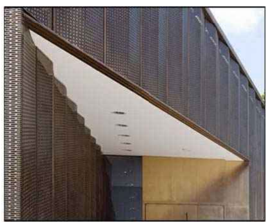
8. FIBRE CEMENT SOFFIT LINING PAINT FINISH: WHITE
